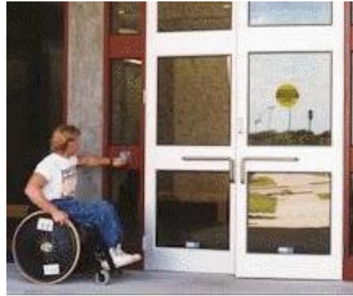
Figure 5: Automatic door opener, with large push button affixed to left of sliding doors.
